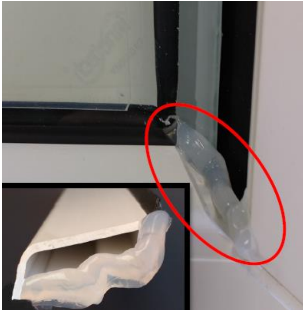
Fig. 3 Add neutral-cure silicone sealant
