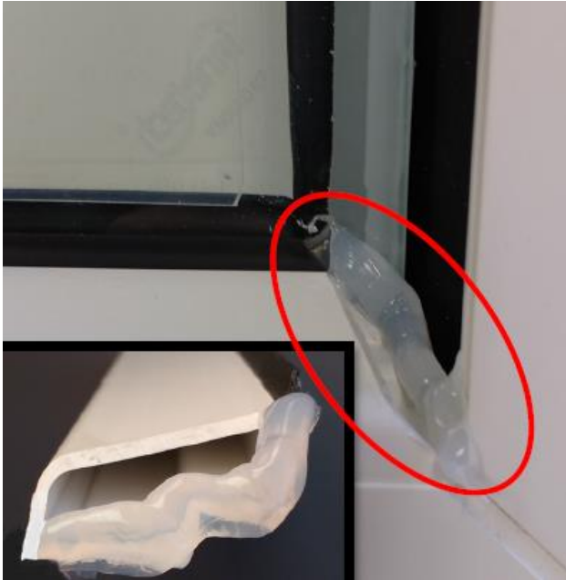
Fig. 3 Add neutral-cure silicone sealant
