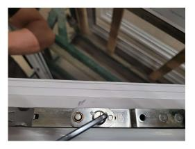
Up - down adjustment of sash at bottom of hinge
