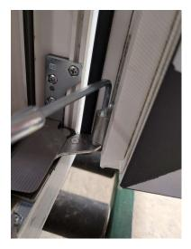
Left - right adjustment of the sash at the bottom of the window
